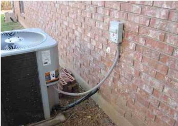
Central heat and air-conditioning are provided by a heat pump, with an air handler located in attic. The heat pump was manufactured in 2014. The air handler was manufactured in 2014.
